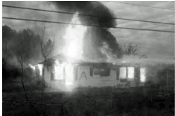
BURNING OF THE OLD DEPOT BUILDING, 2015. PHOTO FROM MELINDA GILBERT VIA FACEBOOK.
